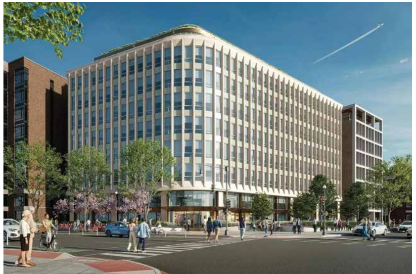
1625 MASSACHUSETTS AVE NW, OFFICE TO RESIDENTIAL CONVERSION
