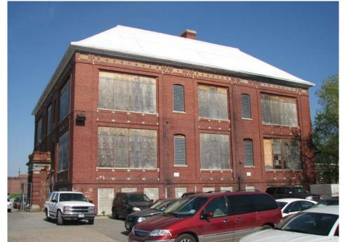
Front (south) elevation of building as seen from Gallaudet Street. The exterior wall system is in generally good structural condition
