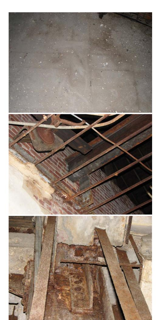
Connection of floor framing as seen at core area of first floor
