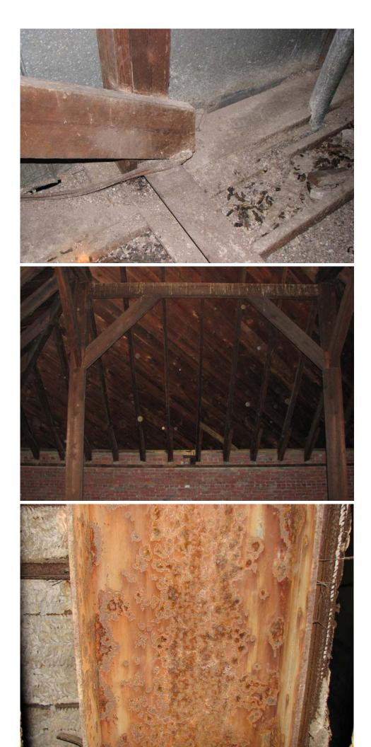
Connection between lateral rafter bracing and steel girder
