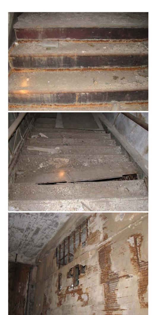
Sectional corrosion at tread to riser connection at stairs. Stairs should be replaced near-term
