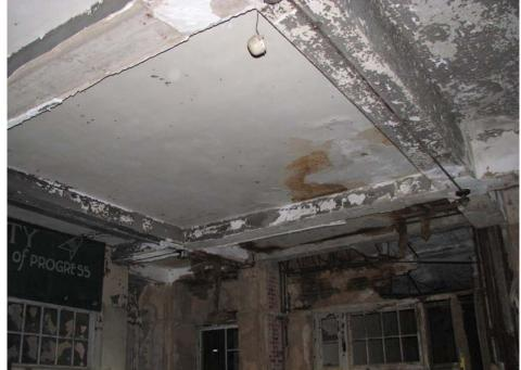
Overview of elevated concrete floor system showing flat panel system supported on concrete encased steel joists. System is in generally good condition
