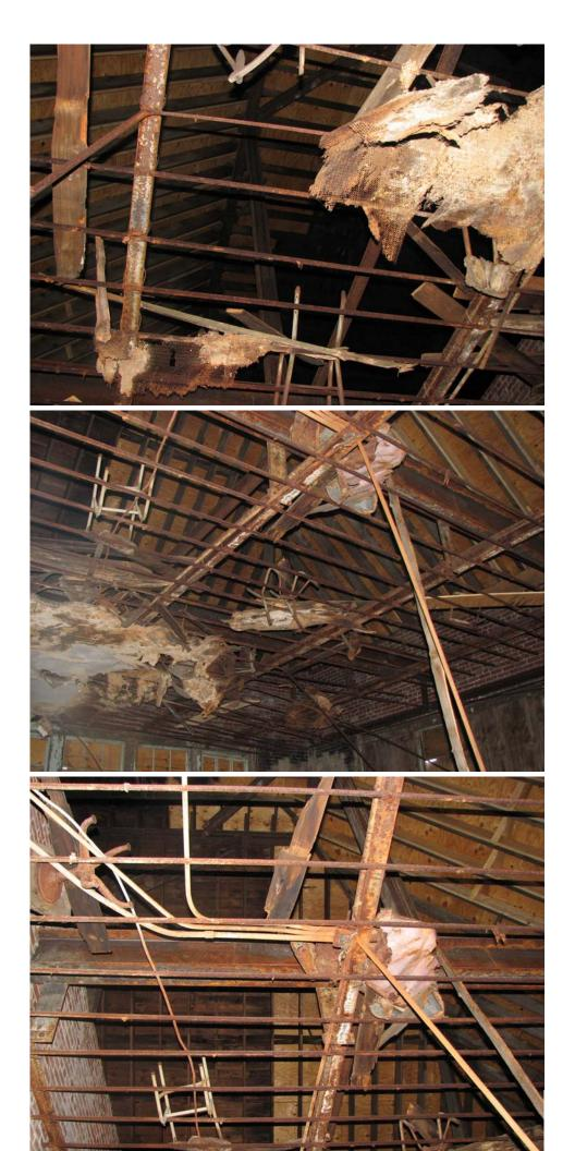
Failure of steel ceiling system above second floor
