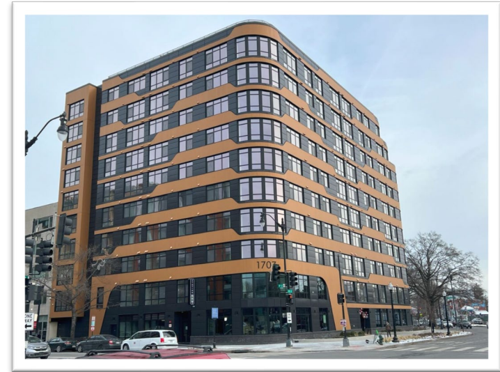
Station U&O is a majority affordable housing complex in the heart of the Shaw neighborhood, delivered by DMPED.
