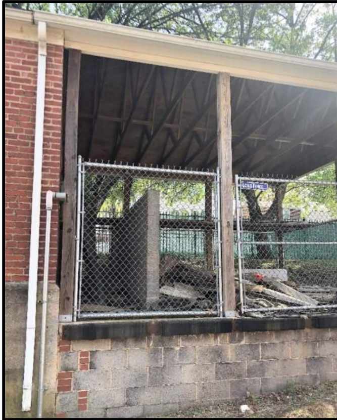
Figure 8 Wood Framing at 1971 Open Storage Shed
