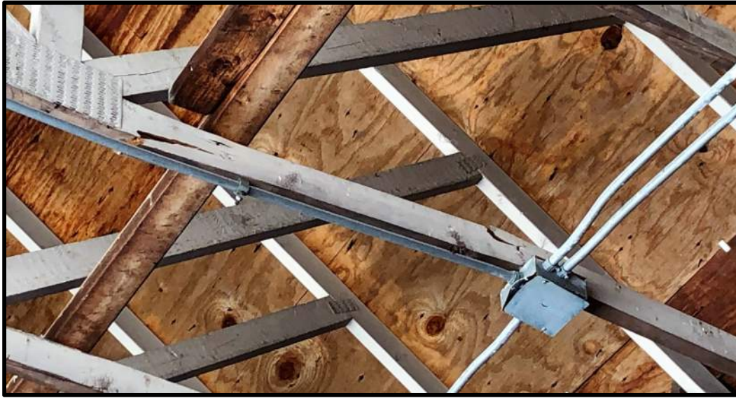
Figure 22 Failed Bottom Chord of Shed Truss
