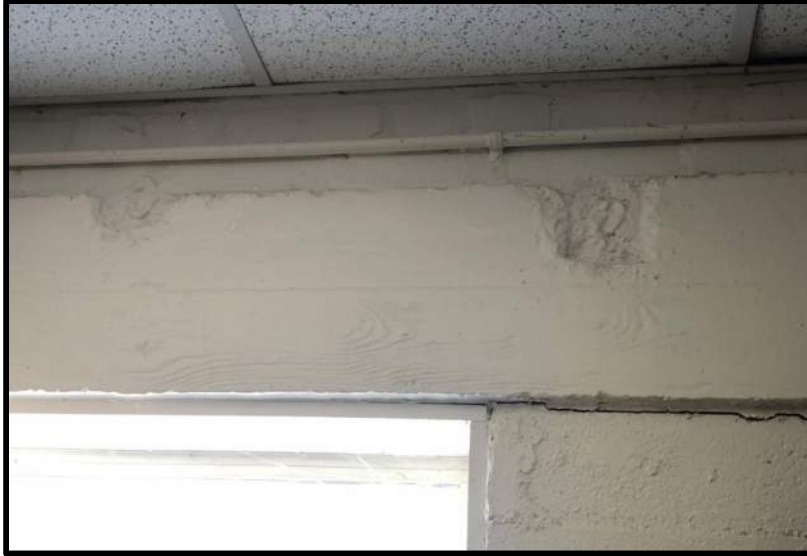
Figure 10 Concrete Spalling at Top of Lintel and Cracking Below
