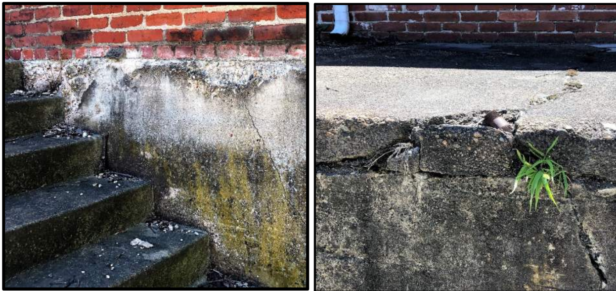
Figure 5 Spalling and Cracks at 1921 Foundation Wall (Left) and Cracking/Spalls at North Platform
