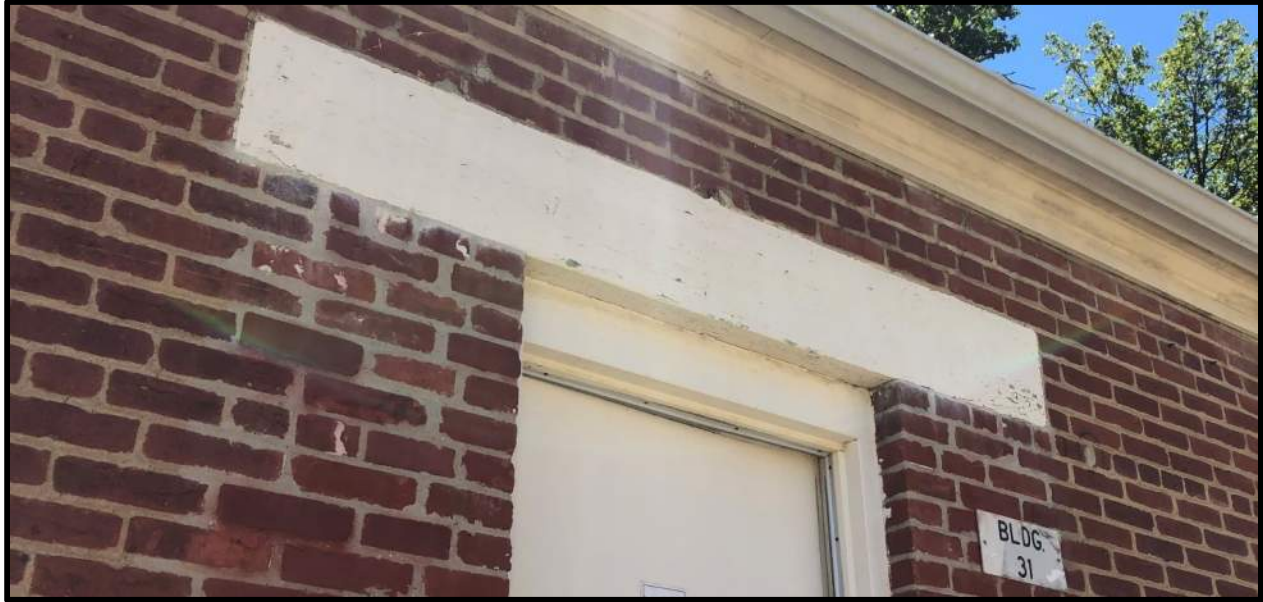
Figure 6 Partially Infilled Opening and Concrete Lintel at Original 1921 Building
