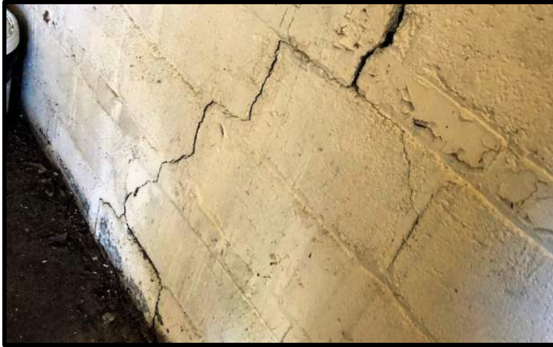
Figure 18 Step Cracking at Masonry Wall
