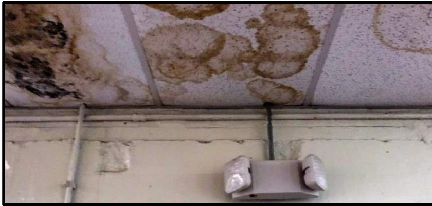
Figure 12 Water Staining at Dropped Ceiling Tiles
