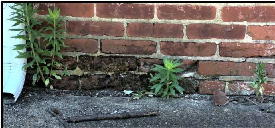
Figure 9 Mortar Loss and Organic Growth Near Grade
