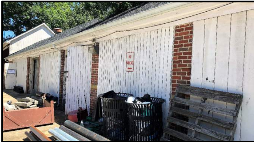
Figure 16 Brick Masonry Piers with Wood Infill at North Elevation
