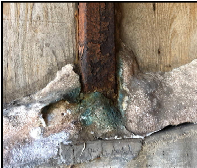
Figure 19 Rust at Base of Steel Tube Column
