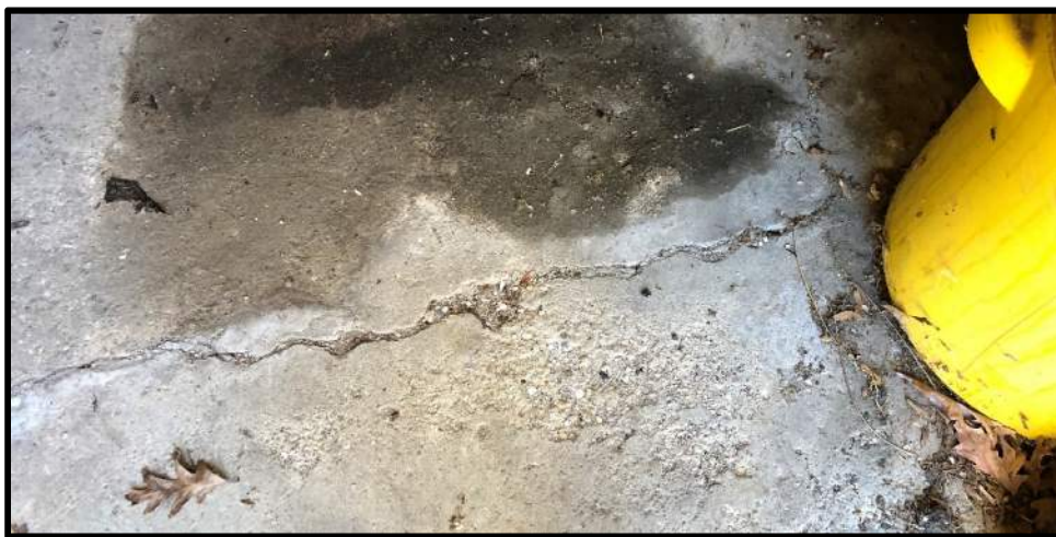
Figure 14 Cracks and Minor Spalling at Slab on Grade
