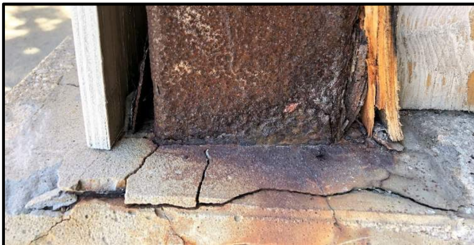
Figure 15 Spalling of Concrete Foundation Walls at Interface with Steel Frame
