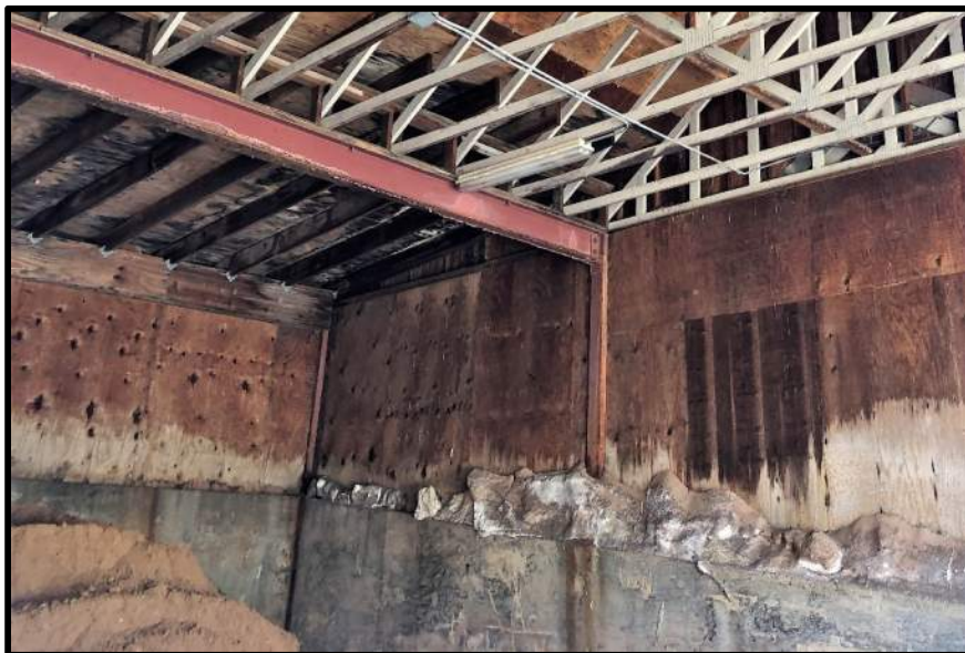
Figure 17 Steel Frame and Wood Infill at Shed Addition
