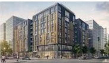
The Elle Apartments 1111 20th St NW (161 Units)
