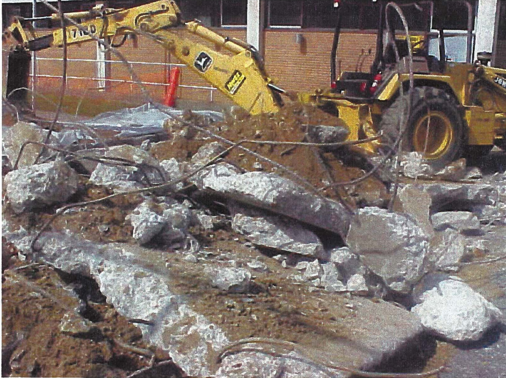
Chevy Chase Branch, DC Public Library – Breaking up concrete pad
