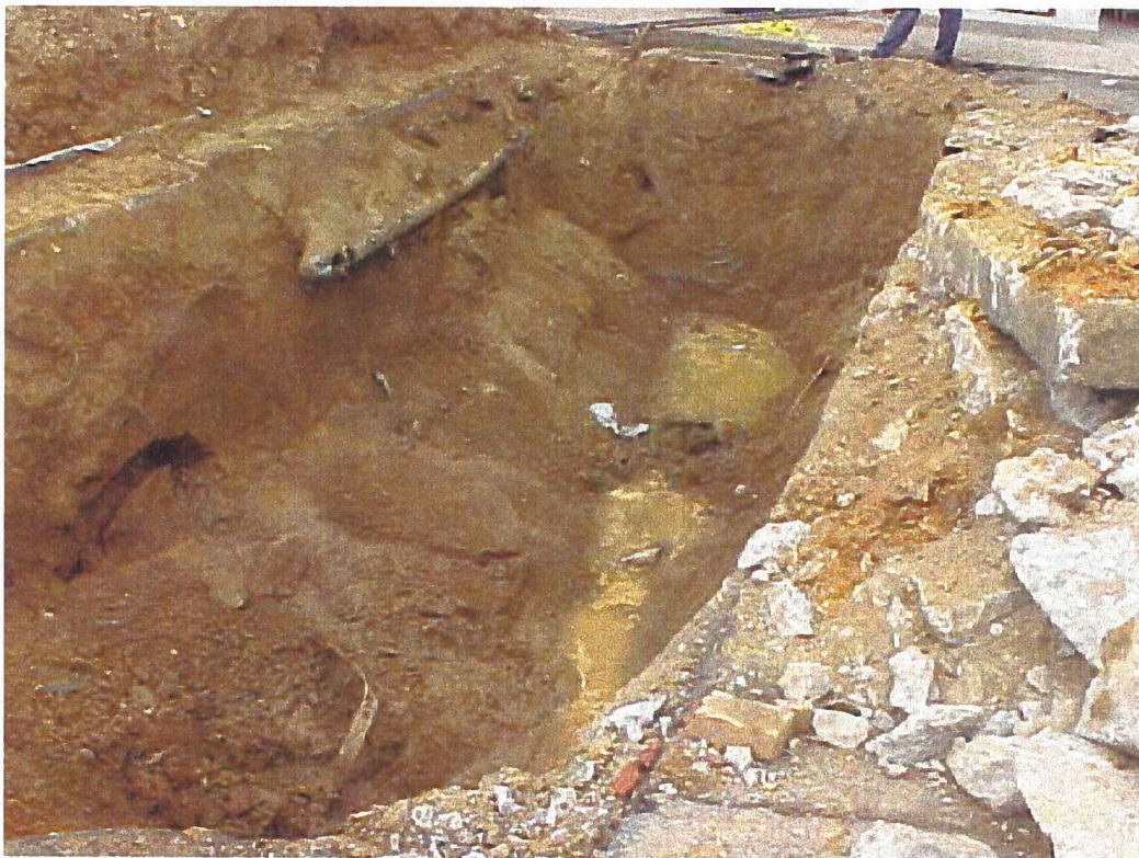
Chevy Chase Branch, DC Public Library – Excavated hole after tank removal
