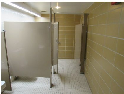
Ceramic Floor Tile (Restrooms)
