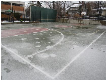
Site Development - Basketball Court - Asphaltic Concrete
