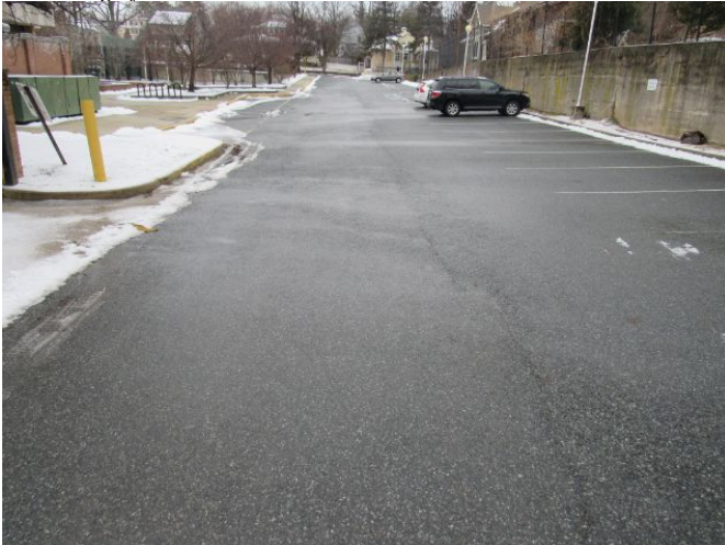
Parking Lot & Roadway - Pavement - Bituminous Parking Lot & Roadway - Pavement - Bituminous March 27, 2021
