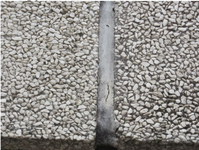
Precast-to-Precast Sealants Precast-to-Precast Sealants March 27, 2021
