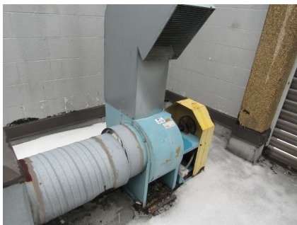
Exhaust Ventilator - Roof - (1,500 CFM)
