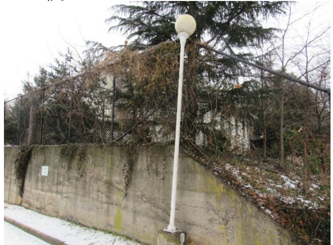
Lighting - Exterior - Pole-Mounted - HID - 12' Lighting - Exterior - Pole-Mounted - HID - 12' March 27, 2021
