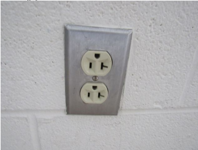
Branch Wiring - Equipment & Devices Branch Wiring - Equipment & Devices March 27, 2021
