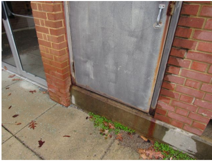
Door Assembly - Single - Hollow Metal (Roof + Generator Enclosure)
