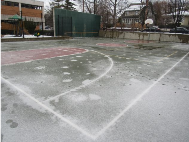
Basketball Court - Asphalt Surface will Exceed Life - Exterior Basketball Court - Asphalt Surface will Exceed Life - Exterior March 27, 2021
