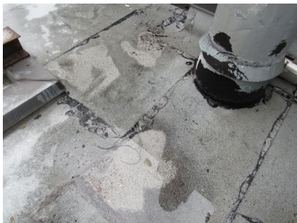
Modified Bitumen Roof
