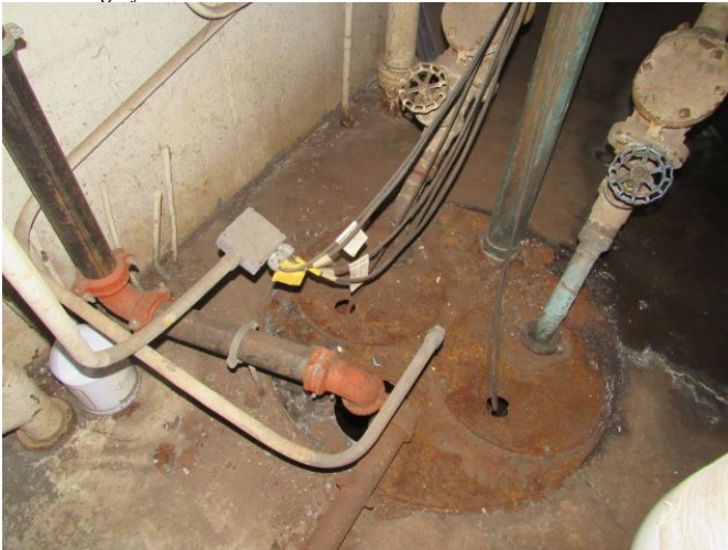
Sewage Ejector Pumps - Duplex Sewage Ejector Pumps - Duplex March 27, 2021
