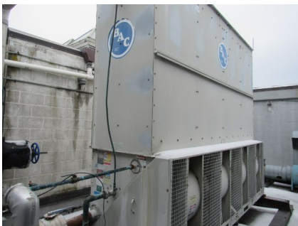
Cooling Tower - Galvanized Steel - 107 Ton
