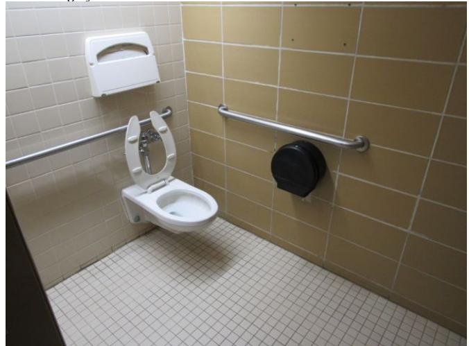
Ceramic Wall Tile (Restrooms) Ceramic Wall Tile (Restrooms) March 27, 2021
