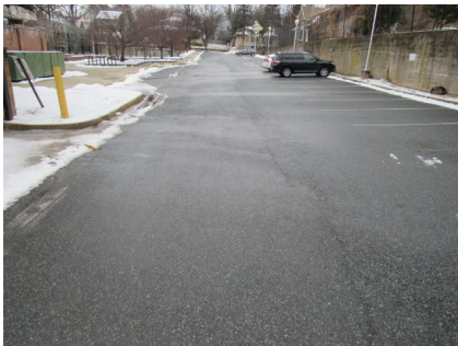
Parking Lot & Roadway - Pavement - Bituminous
