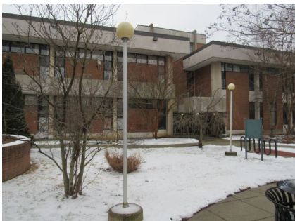
Lighting - Exterior - Pole-Mounted - HID - 10'
