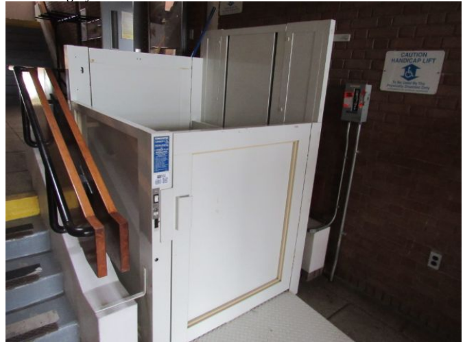
Wheelchair Lift - 750lb (# 1) Wheelchair Lift - 750lb (# 1) March 27, 2021
