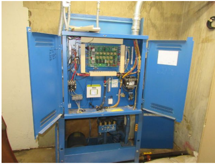
Hydraulic Elevator
