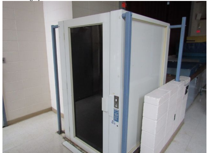
Wheelchair Lift - 750lb (# 2) Wheelchair Lift - 750lb (# 2) March 27, 2021
