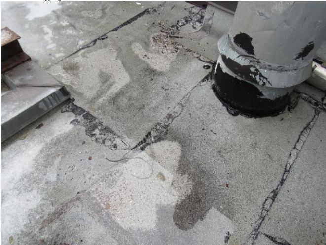
Modified Bitumen Roof Modified Bitumen Roof March 27, 2021
