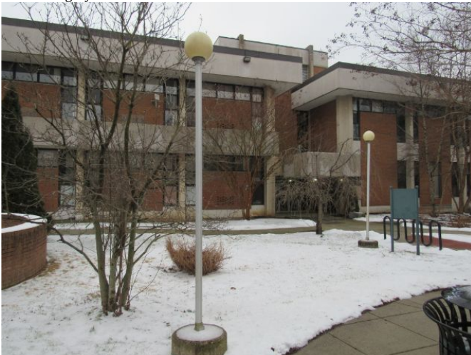
Lighting - Exterior - Pole-Mounted - HID - 10' Lighting - Exterior - Pole-Mounted - HID - 10' March 27, 2021
