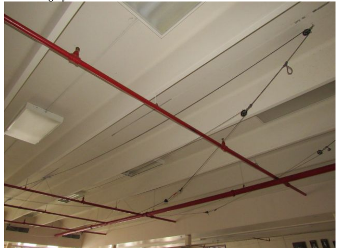
Concrete Superstructure Concrete Superstructure March 27, 2021
