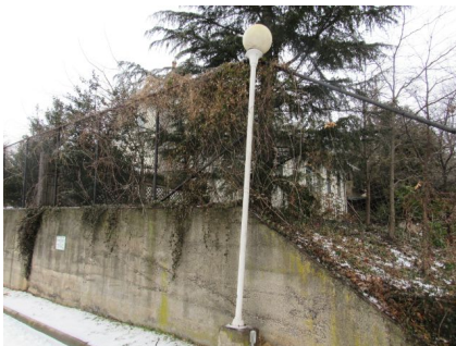
Lighting - Exterior - Pole-Mounted - HID - 12'
