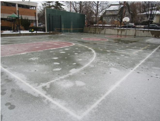
Basketball Court - Color Coat Faded - Exterior Basketball Court - Color Coat Faded - Exterior March 27, 2021
