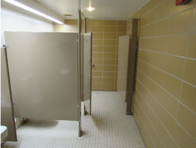
Toilet Partitions - Painted Steel Toilet Partitions - Painted Steel March 27, 2021
