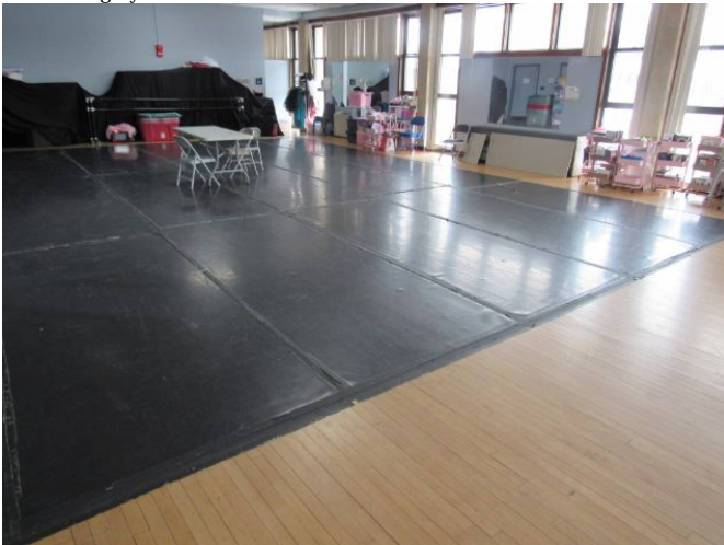
Wood Flooring - Pre-School Play Room Wood Flooring - Pre-School Play Room March 27, 2021
