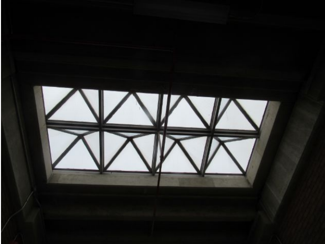
Skylight Skylight March 27, 2021
