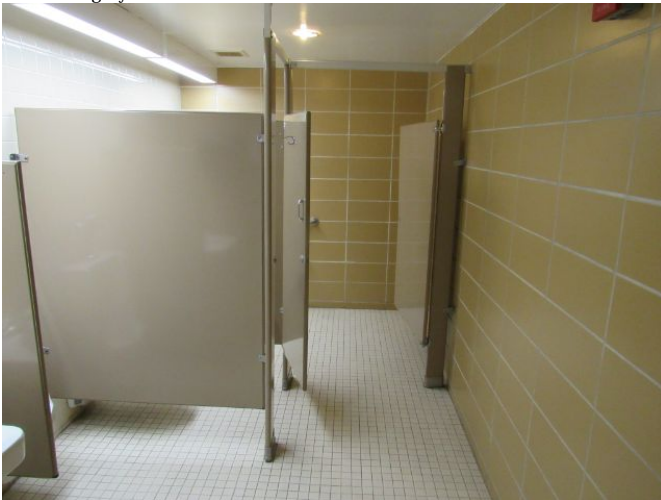
Restroom Fixtures - Multi-Stall Restrooms Restroom Fixtures - Multi-Stall Restrooms March 27, 2021
