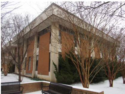
Exterior Architectural Elements - Precast Concrete
