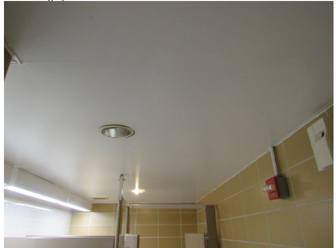
GWB Ceiling System - Painted GWB Ceiling System - Painted March 27, 2021
