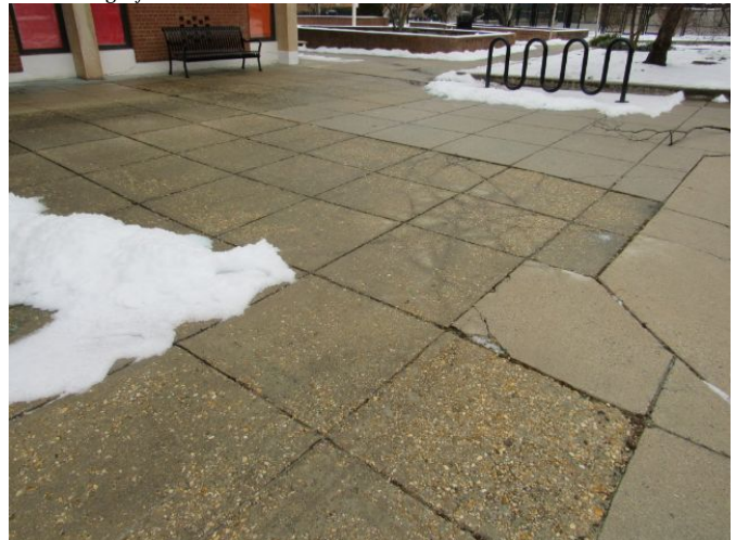
Pedestrian Pavement - Concrete Pedestrian Pavement - Concrete March 27, 2021
