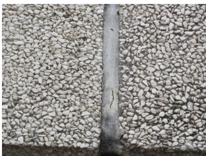
Precast-to-Precast Sealants
