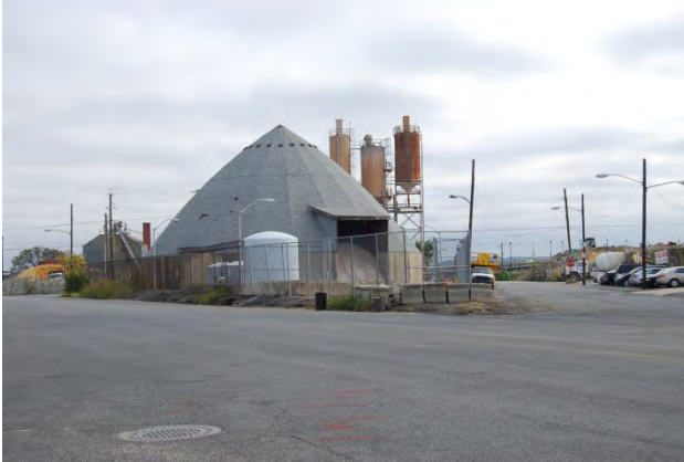
Figure 3-4: Road sand/salt storage facility, located at Potomac Avenue and Half Street
