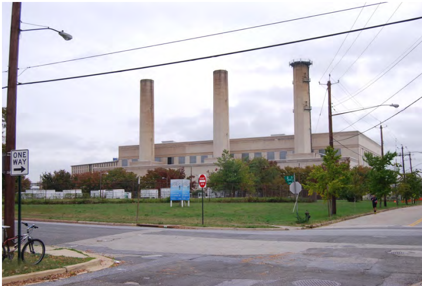
Figure 3-41: PEPCO Power Plant
