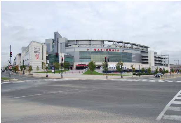
Figure 3-15: Nationals Park, located at South Capitol Street and Potomac Avenue, northeast of the proposed stadium site
