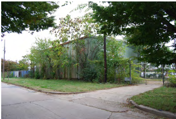
Figure 3-3: Possibly vacant storage building, located at 1 st and S Streets
