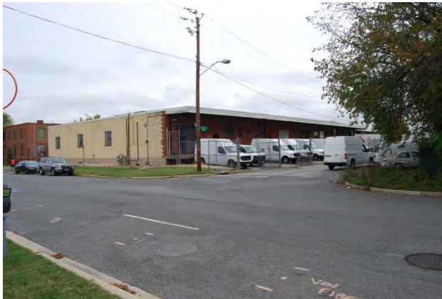
Figure 3-6: Commercial bakery, located at the corner of 2 nd and R Streets
