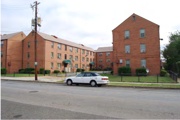
Figure 3-11: Medium-density housing, located on 2 nd Street north of Q Street, north of the proposed stadium site
