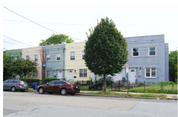
Figure 3-51: Brick rowhouses at 2nd and Q Streets Source: AECOM
